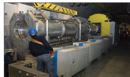
The magnetic horn being installed in the CNGS target chamber.
